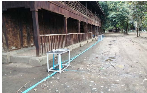
ER 4 Installation of Hand Washing Stations at St. Joseph Quarantine Center.
