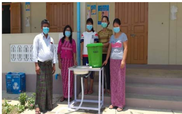
ER 7 Installation of Hand Washing Station in Bhamo Parish Community
